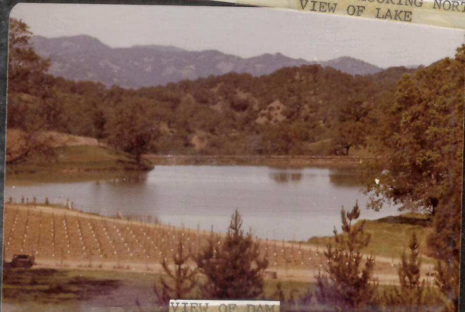
VIEW OF DAM
